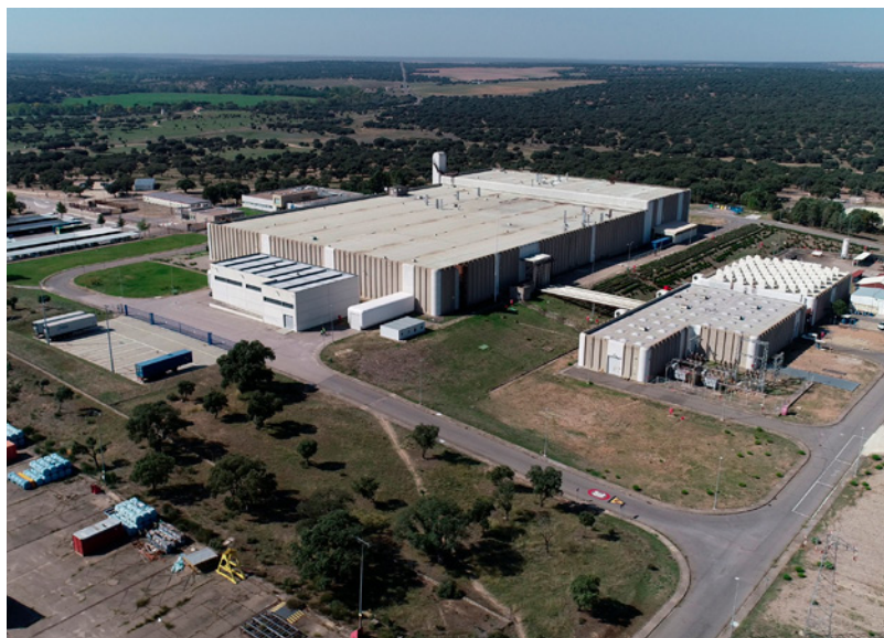
Enusa Juzbado Facility
