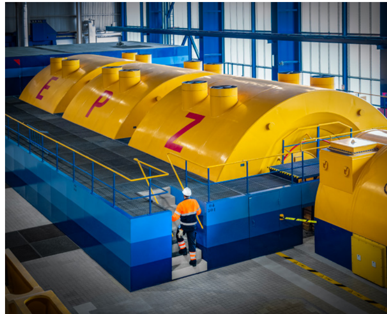
RRF EPZ turbine
